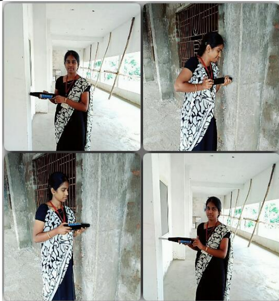
Figure 2.7 Taking reading of column of U Block using Rebound Test Hammer
